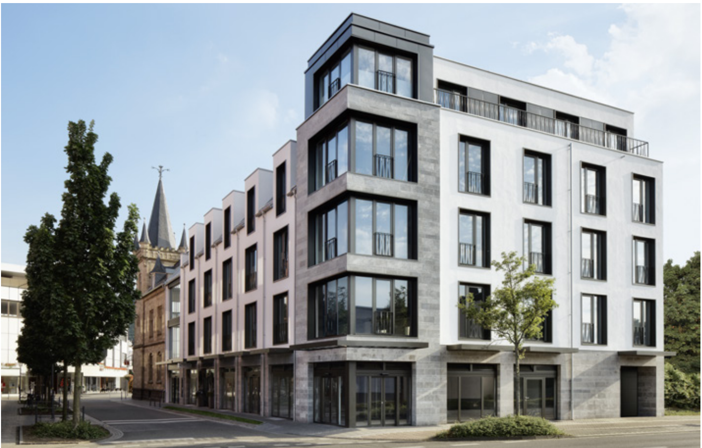
Office building, Bad Neuenahr-Ahrweiler, Germany
