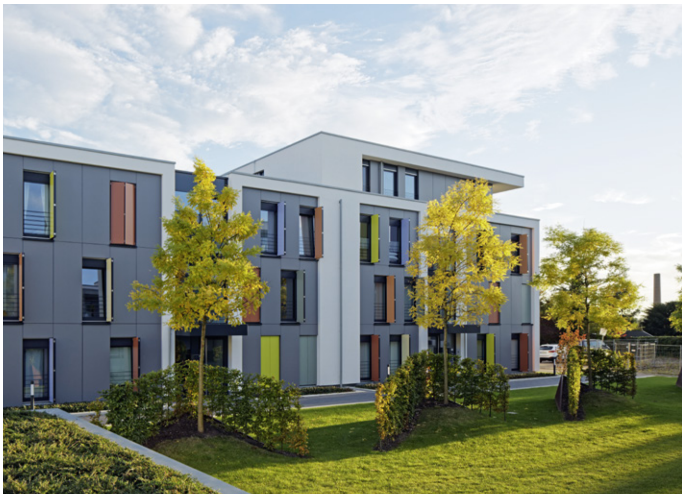
Residential development, Willich, Germany
